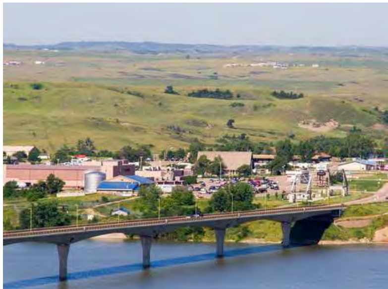
Figure 2.7-2 Four Bears Bridge crossing Lake Sakakawea.
