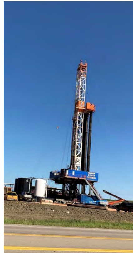
Figure 5.3-1 Typical Drilling Rig
