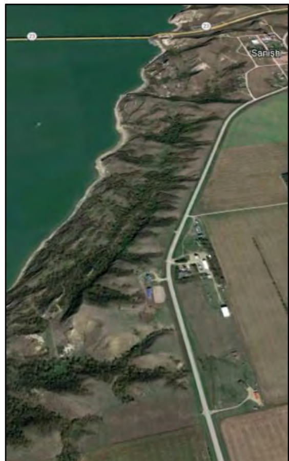
Figure 4.4-5 Aerial of the landslides south of Four Bears Memorial Bridge
