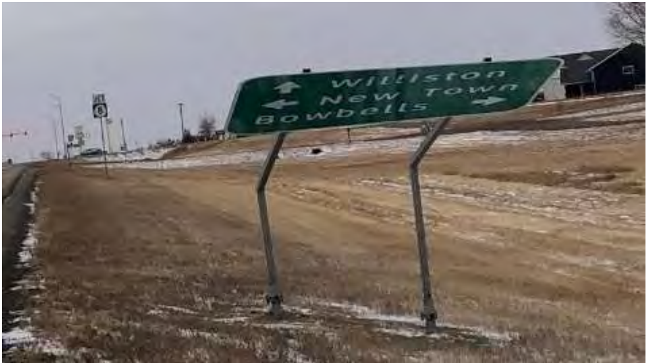
Figure 4.5-3 Recent Wind Damage
