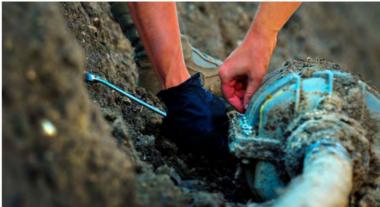
Military personnel splice a cable in the hardened intersite cable system. (Photo credit: Minot Air Force Base)
